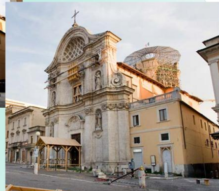
Restoration of Dome
