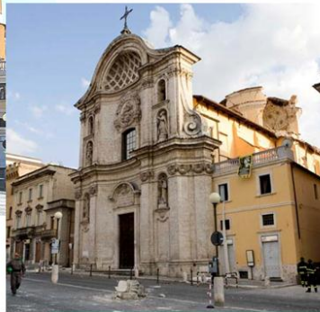
Soon after earthquake Dome ruined
